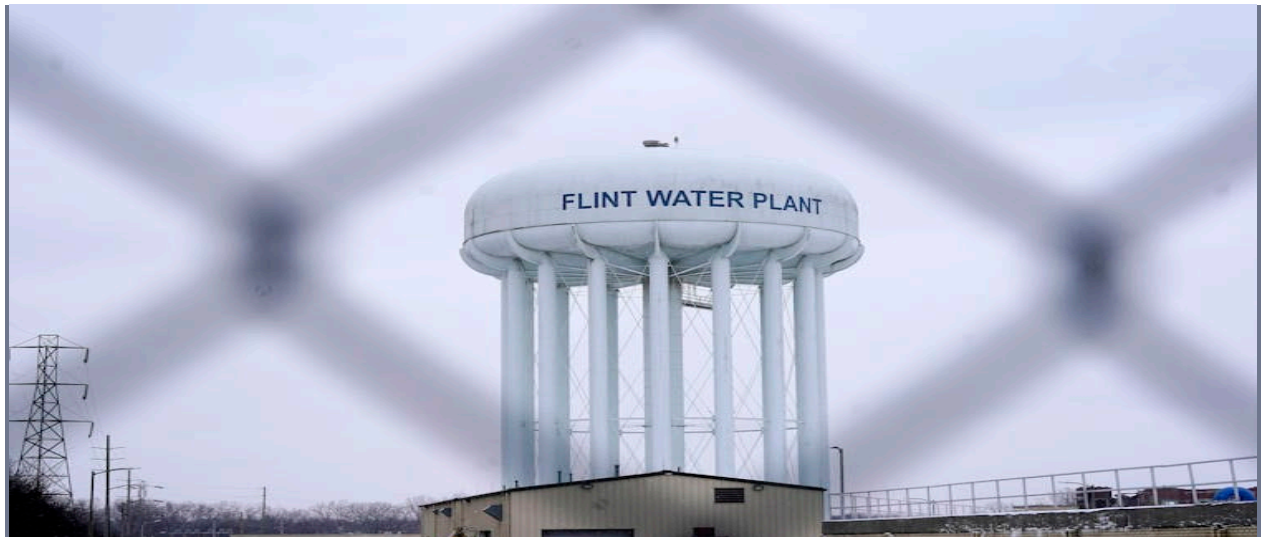
The Flint water plant tower in January 2022 in Flint, Mich. (AP Photo/Carlos Osorio, File)
